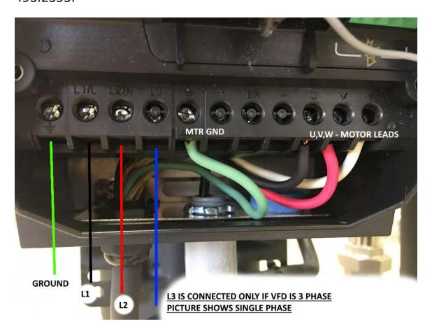
Make note for proper wire gauge based on amp output on side of VFD. Skids with single point entry may have external terminal box AS SHOWN BELOW.
