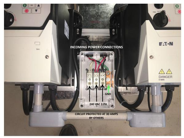
3HP DUPLEX SHOWN WIRE SIZE IN SHOULD BE NO LESS THAN 12 GAUGE RATED FOR 30 AMPS FOR 230VAC SINGLE OR THREE PHASE INPUT.
